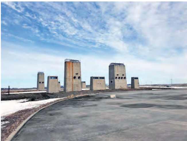
The MSPP generator stacks taken from the top of the heatsink. The taller ones are exhaust with the shorter ones being intakes
